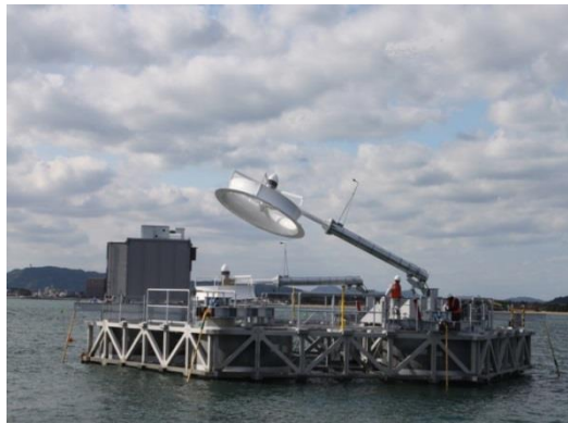
Hakata Bay, Fukuoka City: 18m Hexagon floating body and two 3kW Wind-Lens Turbines (WLT) and 2.0kW Solar Panels (2011.12.4)
