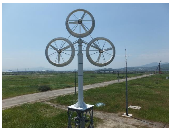
Hibiki-nada, Kita-kyushu City: 9kW Multi-WLT system (2016.3 & 2017.3)
