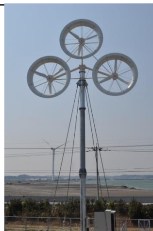
Hibiki-nada, Kita-kyushu City: 9kW Multi-WLT system (2016.3 & 2017.3)
