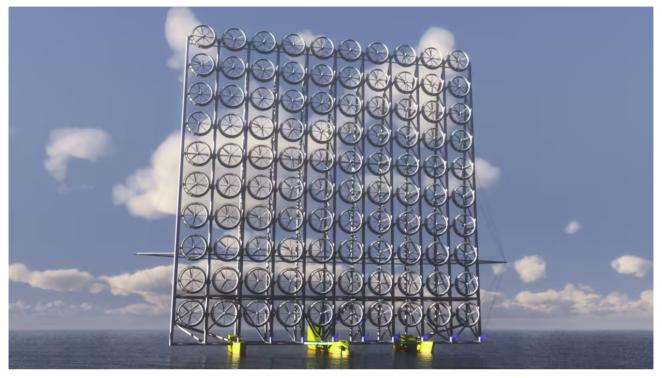
A multi-turbine system can theoretically generate more power than a single-turbine unit of similar size, according to researchers. (Image courtesy of Kyushu University)
